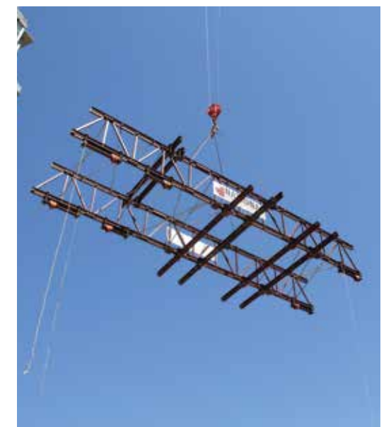
Support Truss Structure Assembly
